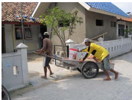
Carrying construction materilas
